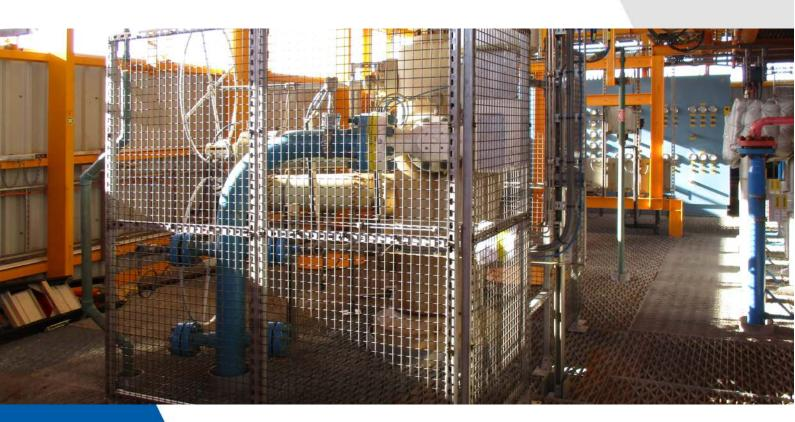
Personal protection panels, also referred to as personal protection (p.p.) are used to protect people from the hot parts of installations. This type of insulation consists of perforated protective caps that are placed directly onto the part using spacers. If it cannot be mounted directly onto the parts, the construction will be self-supporting, even allowing it to shield off entire areas.
